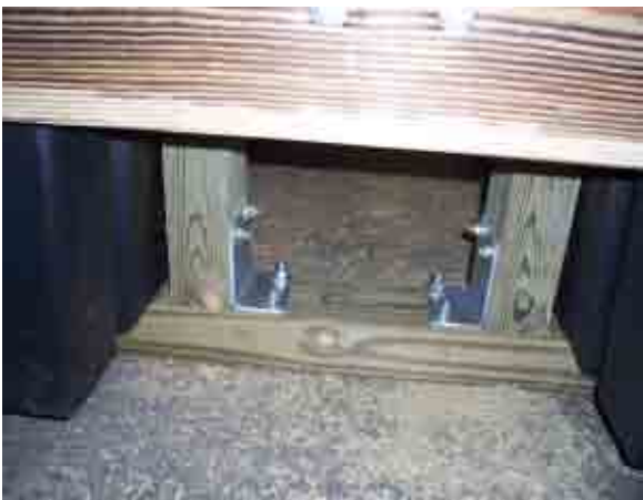
90° JOIST STIFFENER PLATE (6H414) USED FOR BOTTOM SKID PLATE ATTACHMENT
