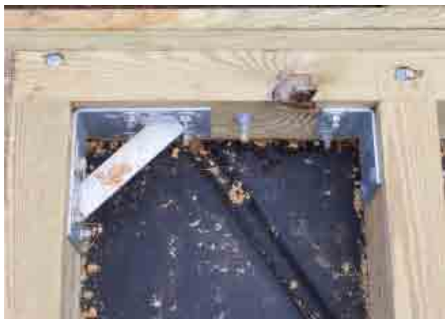
INSIDE CORNER (6H411) & 90° STIFFENER PLATE (6H414)
